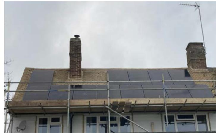
In the end we decided on 25 \* LG 375W full black solar panels with edge inverters and a SolarEdge main inverter. Our house roof has a West/East orientation, so this is how the configuration was installed:
