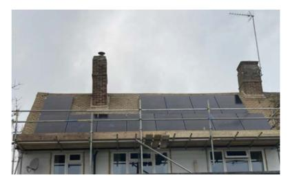
In the end we decided on 25 \* LG 375W full black solar panels with edge inverters and a SolarEdge main inverter. Our house roof has a West/East orientation, so this is how the configuration was installed:
