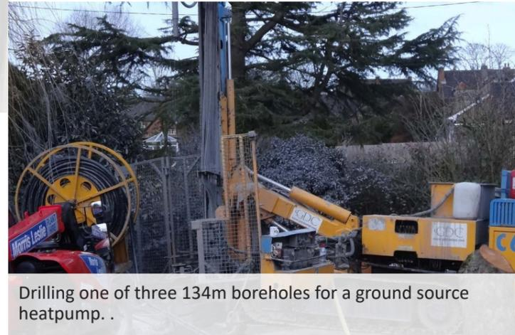
Drilling one of three 134m boreholes for a ground source heatpump. .
