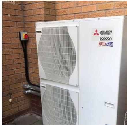
14 kWh EcoDan air source heat pump. These are particularly good units as they continue to perform consistently in sub-zero temperatures.
